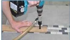
**Step 2** Using a template to stabilize the drill bit, begin slowly drilling with light pressure.
