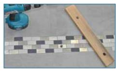
**Step 3** Gradually increase drilling speed and maintain steady pressure until the desired depth is achieved.
