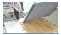
**Step 4** With the saw turned off, place the mosaic sheet, paper side up, on the cement board covered saw tray and align the cut.
