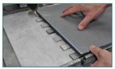
**Step 5** Place the second piece of cement board on top of the mosaic sheet. Cover the portion of sheet that is to be installed (keeper) with the weather-strip side down and against the blade. The board will protect the mounting paper from saw over-spray.
