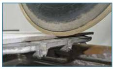
**Step 2** Adjust the blade height so the blade cuts through ½ of the cement board thickness.
