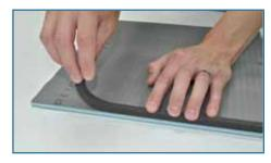
**Step 3** Cut another piece of ½" cement board to a square size that is larger than a sheet of mosaics. Apply a strip of self-adhesive, compressible, foam weather-strip to one edge of the cement board.
