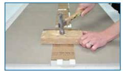
**Step 2** After the installed cement board layer has cured for a minimum of 24 hours, install and grout the tile per the Oceanside Glasstile Installation Guide.
