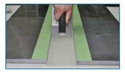
**Step 1** Apply a thin layer (bond-coat) of a recommended thin-set.
