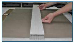
**Step 1** Using a recommended thin-set, install a piece of ¼" or ½" cement board. Use a notch trowel size and cement board thickness that will render the desired substrate depth. Cure a minimum of 24 hours.
