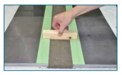
**Step 2** While the bond-coat is still tacky, apply a cement mortar bed (4:1 sand & cement mixture per ANSI A108.1B). Screed the cement mortar bed to the desired substrate depth and cure a minimum of 7 days.
