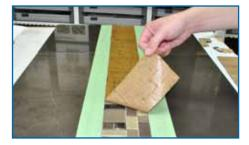
**Step 3** After the cement mortar bed has cured a minimum of 7 days, install and grout the tile per the Oceanside Glasstile Installation Guide.
