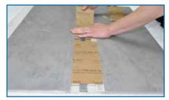
**Step 2** After the build-up layer of thin-set has cured for a minimum of 48 hours, install and grout the tile per the Oceanside Glasstile Installation Guide.
